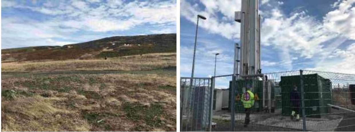
Figure 46 The old landfill surface already looks like the surrounding landscape except the visible gas wells in black (left), the handy landfill gas processing station in Akureyri (right) (credit: Felicitas Schneider)
